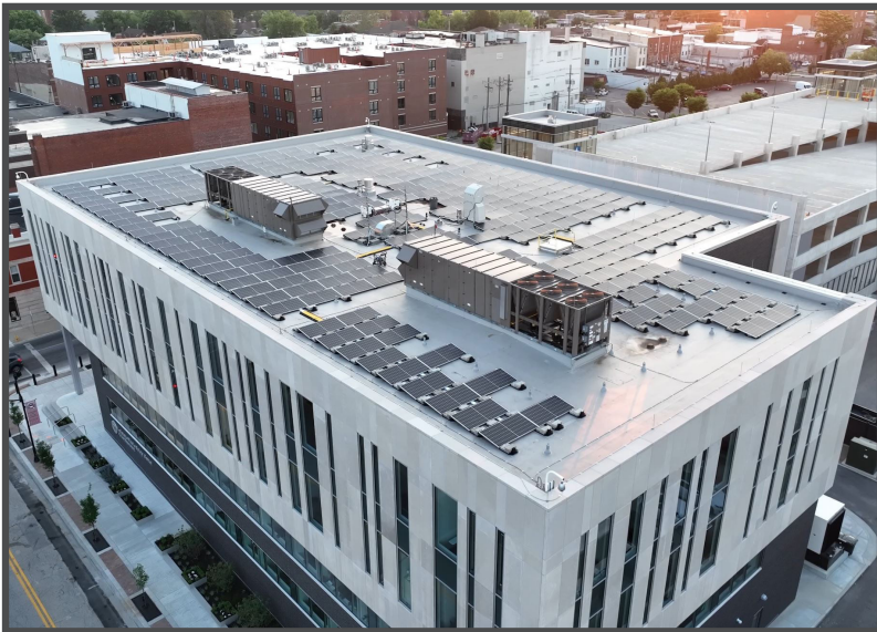
The array of over 200 (80kW) solar panels is estimated to offset energy usage by up to 40%.
