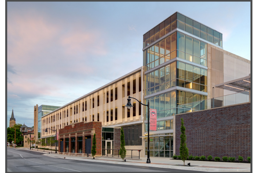
By preserving and recycling the materials from the old building, our construction carbon footprint is reduced.
