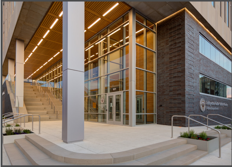
Strategic use of glazing allows this building to reduce artificial lighting loads while also creating inviting and welcoming spaces for the public.
